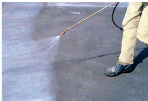
**Curing compounds** are used to minimise the loss of moisture from the concrete slabs during the hydration period maximising density and durability and minimising the chance of cracking, and curling. There are several types of curing compounds available including Hydrocarbon Resin, Wax Emulsion and Acrylic emulsion which meet the Australian Standard AS3799.
