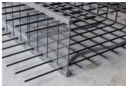
**Stremaform®** formwork elements for working joints divide large structural components into individual concreting sections. The prefabricated elements are used as permanent formwork in floor slabs, ceilings and walls. Stremaform® formwork guarantees a rough surface. Shear forces are transmitted via this working joint. The formwork lies between the continuous reinforcement layers so that there is no need to interrupt the reinforcement.
