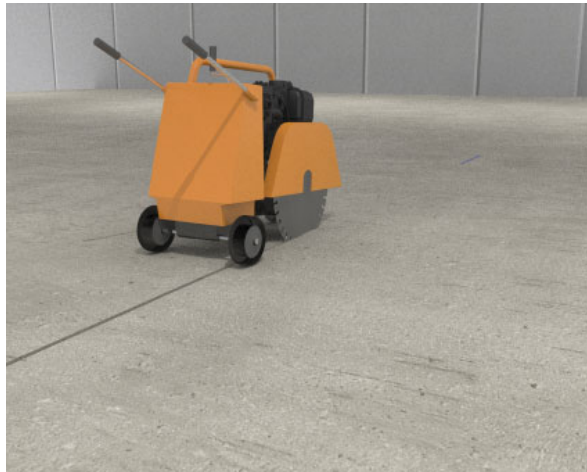
Saw cut the slab to create the contraction joint
