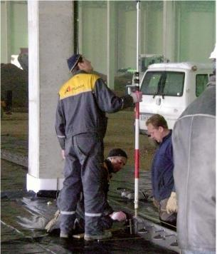
If required by the design, 'X' or 'T' junctions should be placed according to the required layout and set to the correct height using a laser level or equivalent.
