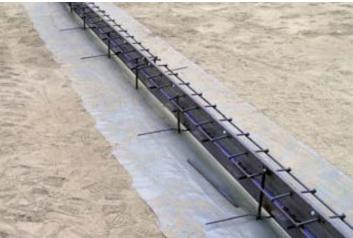
4. As an alternative; TFX Installation Device can be used for TERAJOINT® installation. TFX is a simple to use 'jack' that not only fully supports the floor joints during set-up and pouring of concrete but also allows precise adjustment of the joint height which is critical for high-quality concrete floor slabs. The only TFX is recommended for installation of TERAJOINT® on top of insulation material (for example at cold storage projects). TFX Installation Device is a re-usable item.
